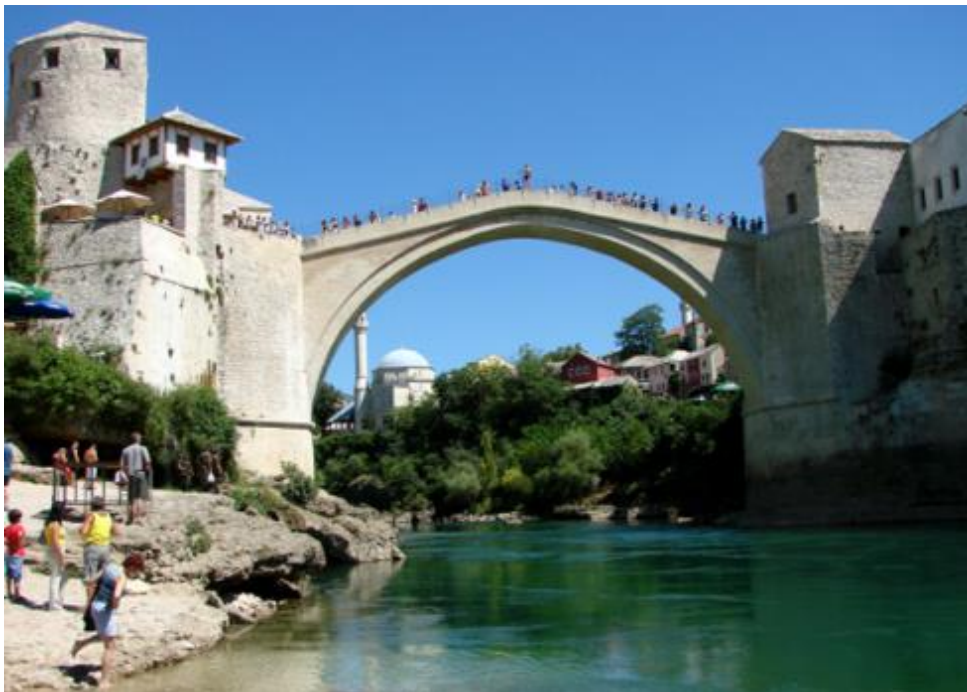
Figure 41 The Rebuilt Mostar bridge
