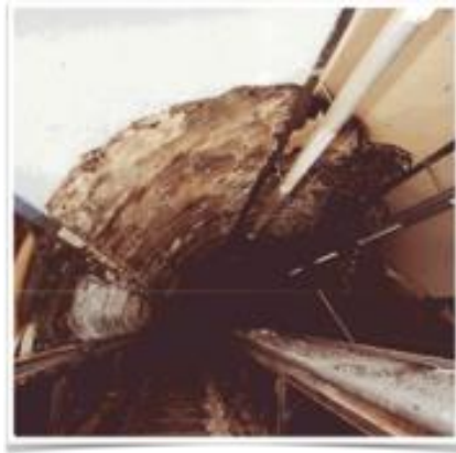
Figure 17 King's Cross Piccadilly Line escalators in 1987 after the fire
