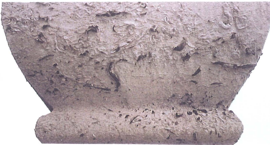
Figure 5.16 Blackened shells and fine crust growth on shells protruding from the stone surface.
