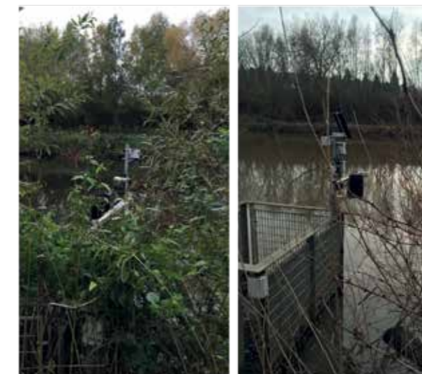
▲ Figure 6. Seasonal variation and harsh weather conditions may cause issues to citizens in accessing sensors as well as affect sensor readings. This needs the physical presence and availability of trained personnel and sensor developers. The image shows the same sensor at different times of the year (left - March, right - November).
