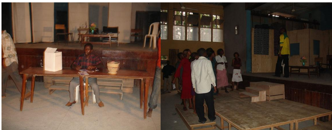
Fig.3: Front of stage before (left) and during (right) construction.
