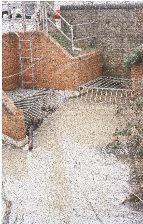
Plate 4-3 Storm water entry through side-weir into flood by-pass channel
