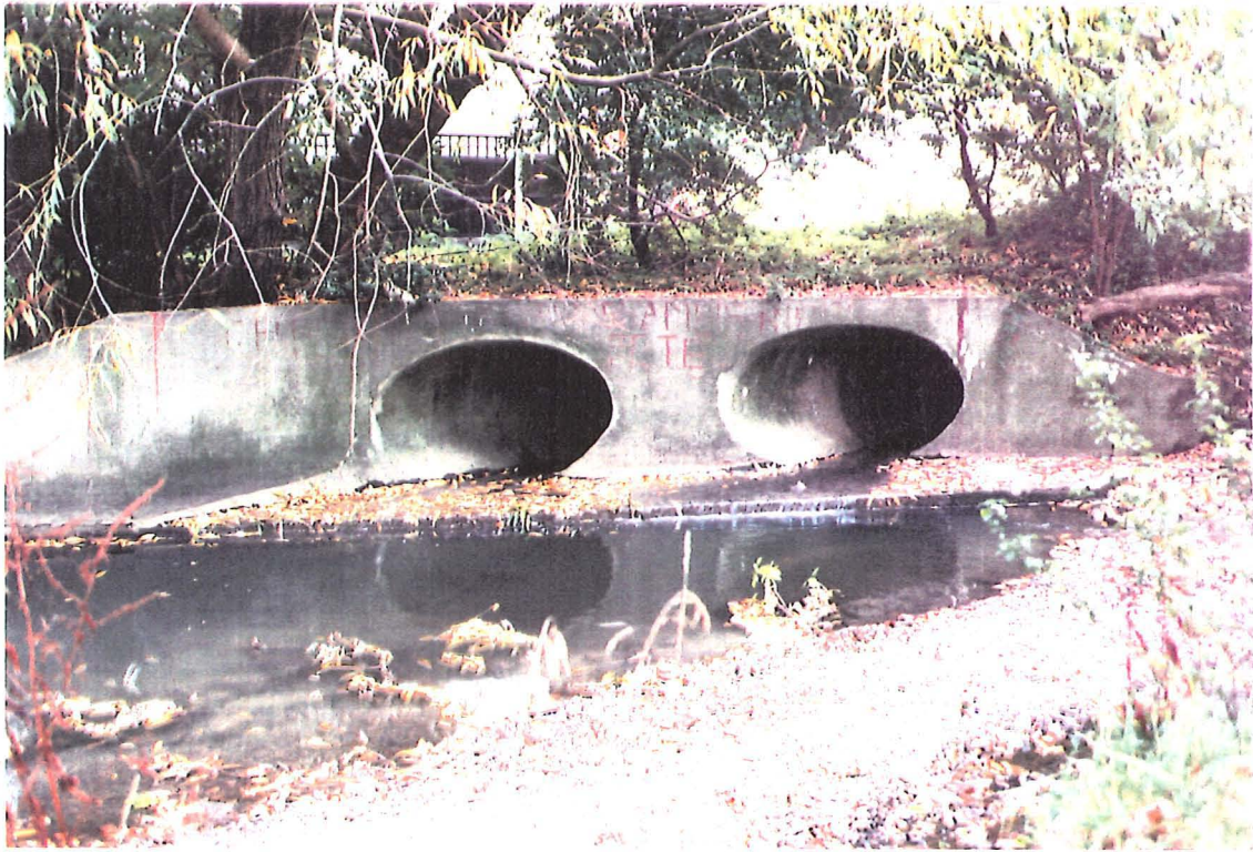
Plate 3.4: Site LD, two combined sewage discharge pipes at Arnos park.
