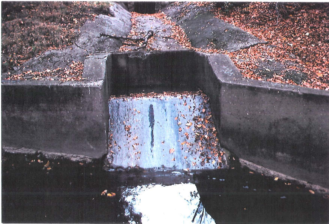
Plate 3.2: Site LB, the combined sewer at Waterfall Walk.
