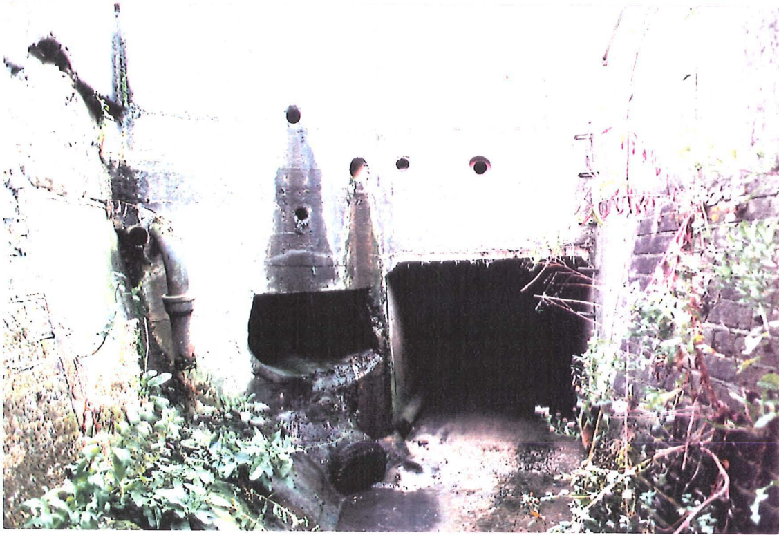
Plate 3.1: Site LA, the combined sewers at New Barnet.
