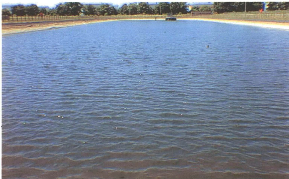
Figure 2.5: View along the length of the Mayfield Farm Balancing Pond; aerators not operational
