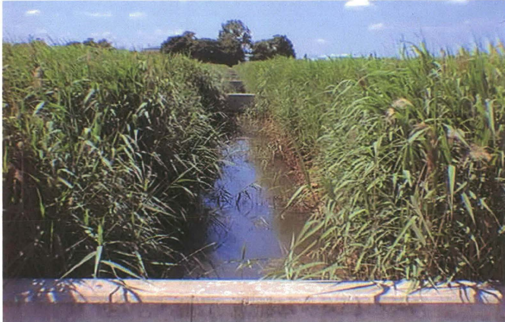
Figure 2.6: View across the sub-surface flow reedbed system showing the open water channels located between the beds
