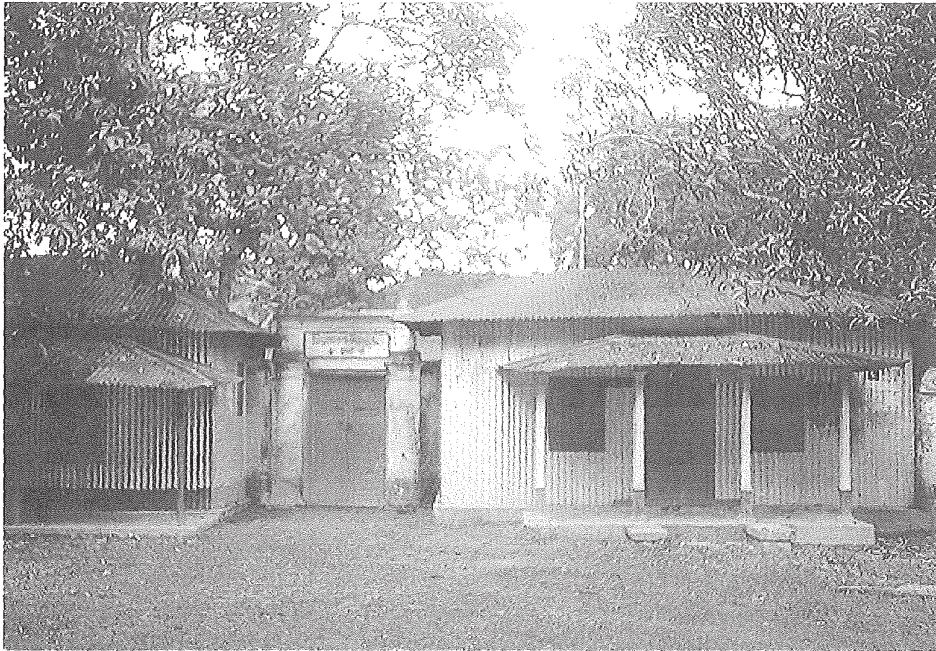
(a) A BC (brick floor, corrugated iron (CI) sheet wall) house (Tangail)
