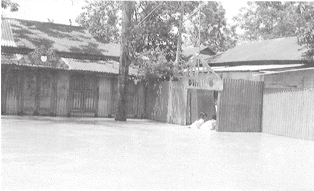
(a) An MC (Mud floor, CI sheet wall) house flooded by 1988 flood (Tangail)
