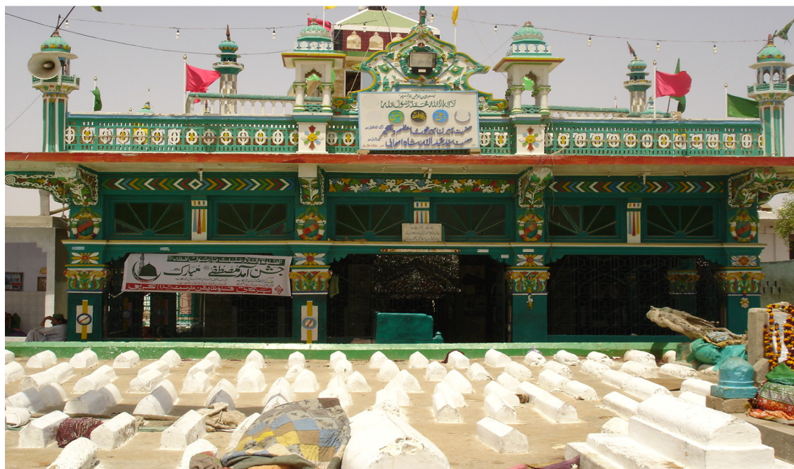
PICTURE II: VIEW FROM THE FRONT COMPOUND. THE MIDDLE SECTION HAS THE ENTRANCE TO THE SACRED DURGAH
