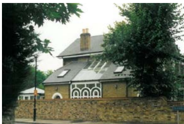
Image 96: After the work was done
