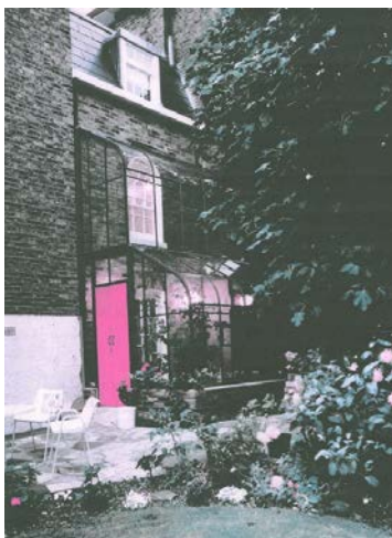
Image 134: A double height conservatory at the rear during the day
