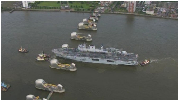
Image 141: The Thames Barrier with its man-made islands that enable large ships to pass through
