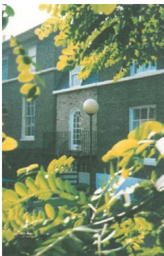
Image 131: After a French window and external stair had been added to 'The Little House'
