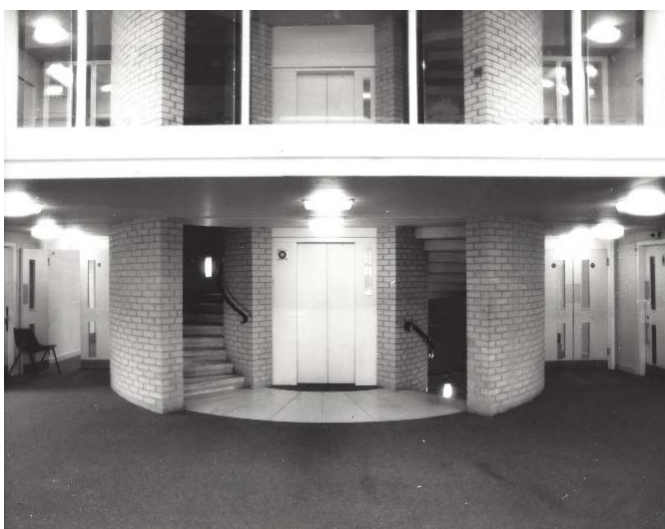
Image 85: When complete with the lift, seen from the central meeting space at ground floor
