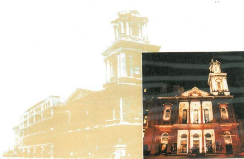
Image A63: City Temple: front elevation before and after it was cleaned and repaired
