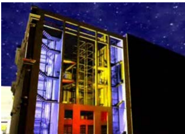
Image A69: The south elevation with its very contemporary glazed wall and visible lifts and stairs
