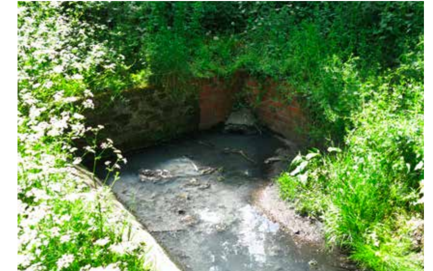
The alternative source at The Green, Houghton Regis
