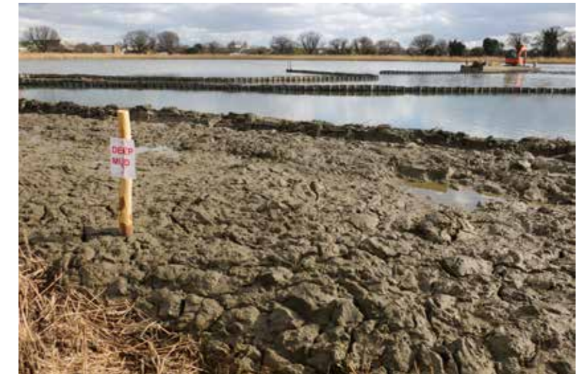
Habitat creation works in progress
