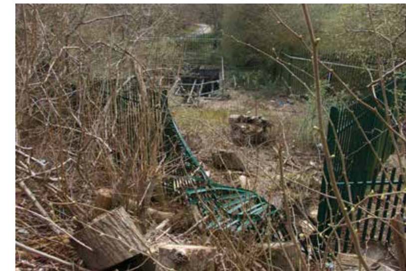
Derelict filter beds outside Luton
