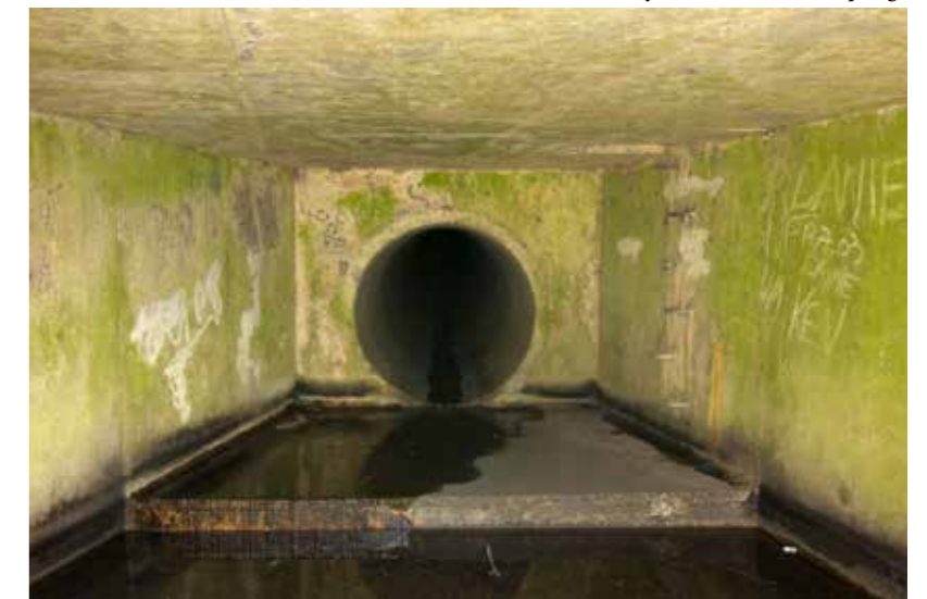
Culvert at the source of the River Lea, Five Springs
