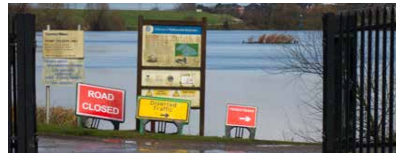
Entrance to the Low Maynard Reservoir
