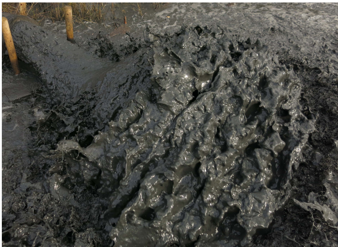
Dredging recharge in operation, Loompit Lake site. February 2015. Copyright Simon Read
