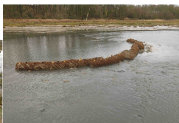
Holding pen at discharge point Coir bund at upper channel Single coir log in small channel February 2015. Copyright: Simon Read
