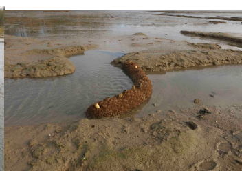
Holding pen at discharge point Coir bund at upper channel Single coir log in small channel February 2015. Copyright: Simon Read
