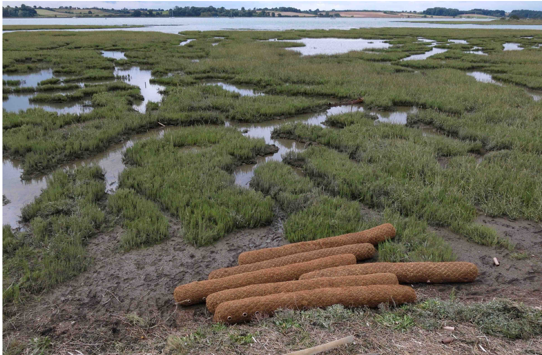
Coir Logs to be located on the western site. 18 th August 2014. copyright: Simon Read
