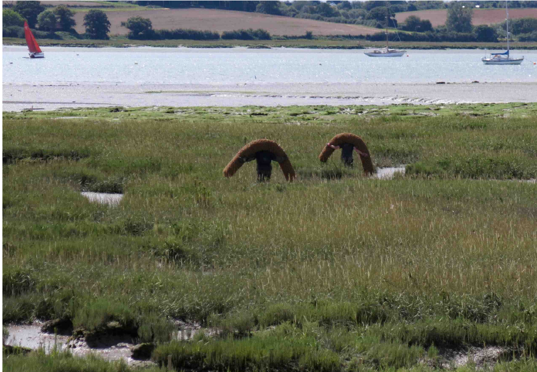
Carrying Coir Logs over the western site: 19 th August 2014. Copyright: Simon Read
