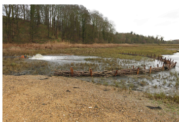
Holding pen at discharge point Coir bund at upper channel Single coir log in small channel February 2015. Copyright: Simon Read
