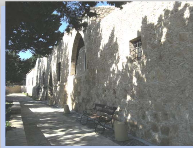
The perimeter wall with the entrance that separates the monastery from the park.
