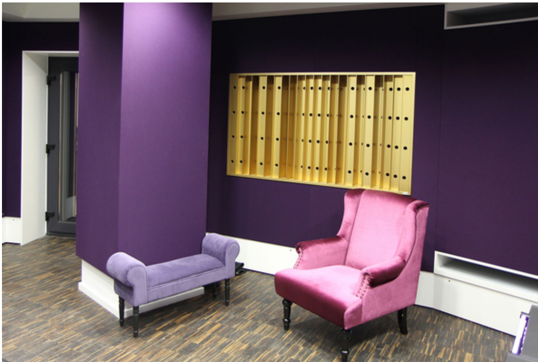
Figure 14: Helmfusor implementation at the back of the large studio of SAE Berlin (opened mid-2016). Photo: SAE Institute GmbH.
