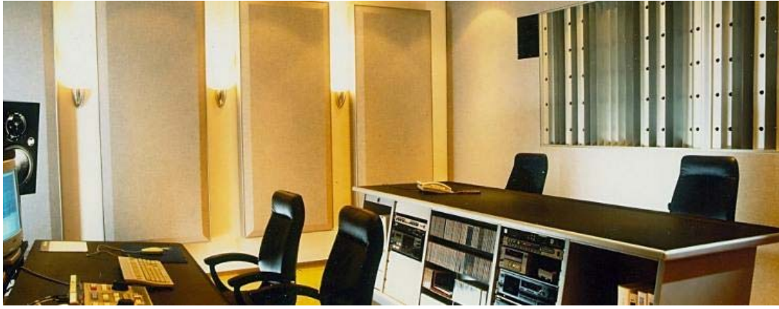
Figure 13: Bevelled broadband absorbers in the back and Helmfusors (see next section) on the right of the picture at a TV studio in the Sendezentrum München. Although these absorbers are only 12cm deep they absorb sound as efficiently as 20cm deep absorbers. Photo: Sendezentrum München (SZM).
