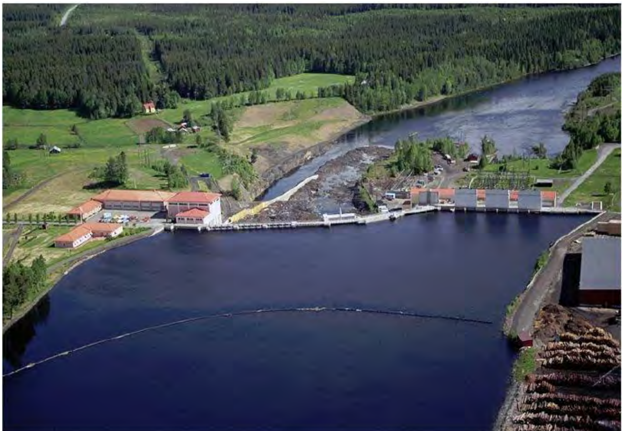
Figure A-8 Construction site in Sweden
