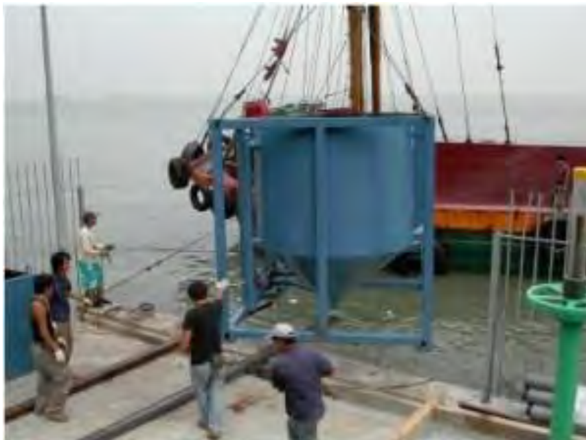
Figure A-5 Transportation of the WetSep by Barge
