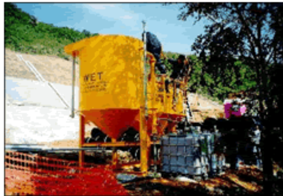
Figure A-2 Installation of WetSep Filtration System for effluent quality control
