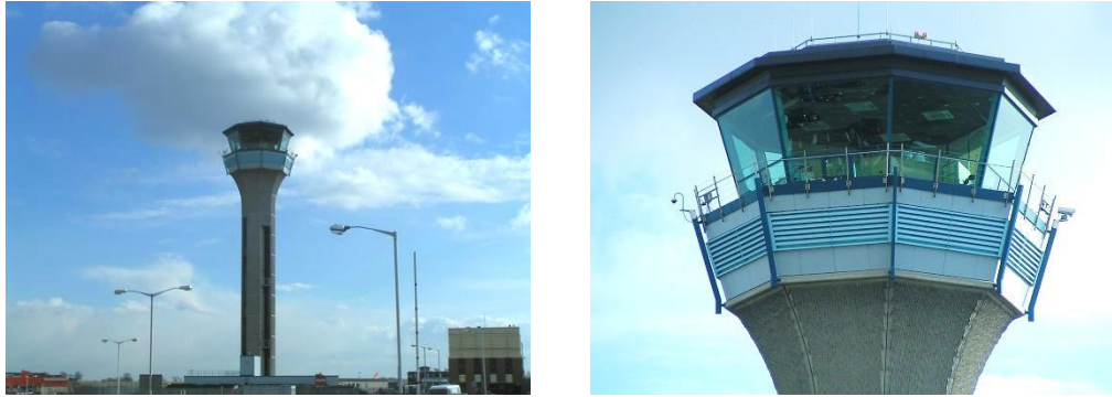
Figure 1 Luton Airport Control Tower
