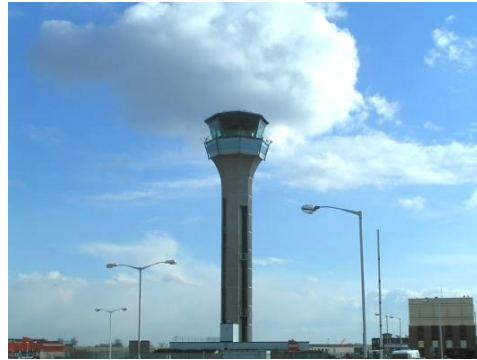
Figure 3- 5 : Control Tower at Studied Airport 8
