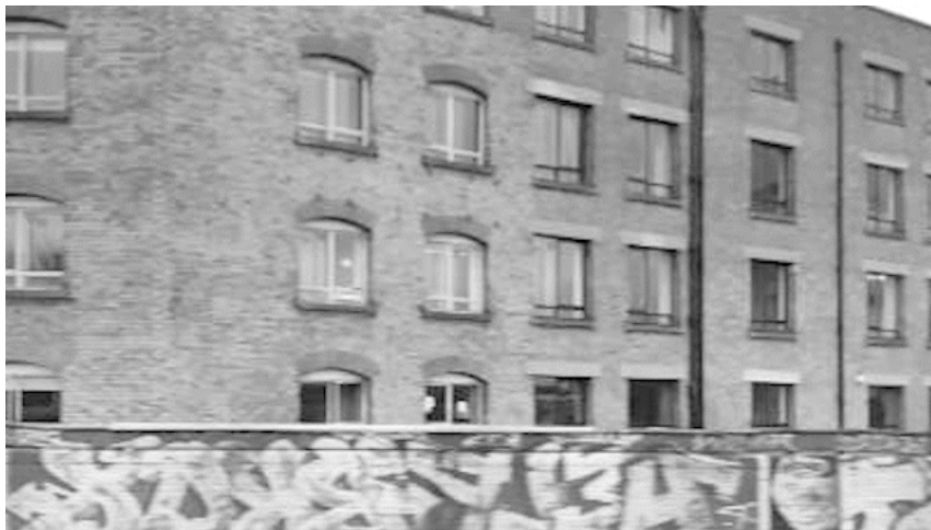
Figure 35. Example of a moving background with no foreground subject.
