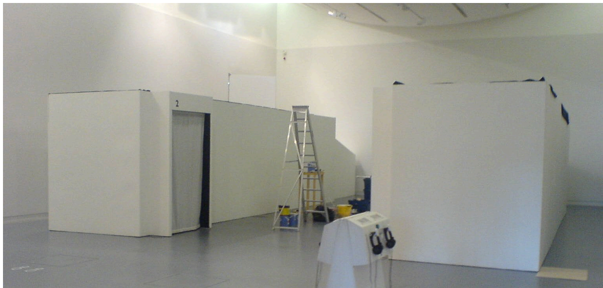
Figure 3. Two Remote Dancing corridors being installed at Aberystwyth Arts Centre, Wales, 2007
