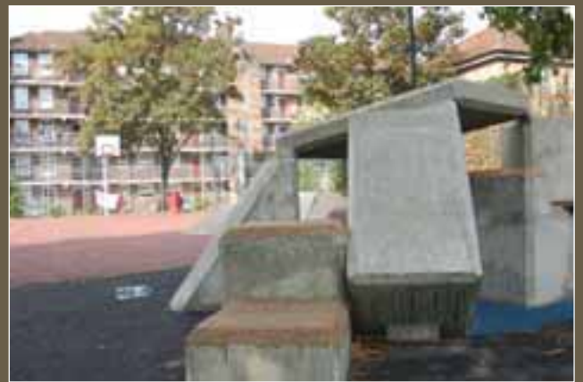
Informal seating/shelter structure.
