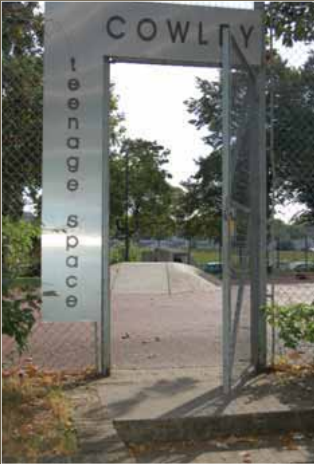
Entrance to Teenage Space: high quality design and specification.
