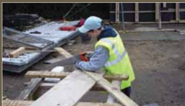
At Spa Fields, the employment on site of local young people was just one of the many means by which this group became actively involved in the project.
