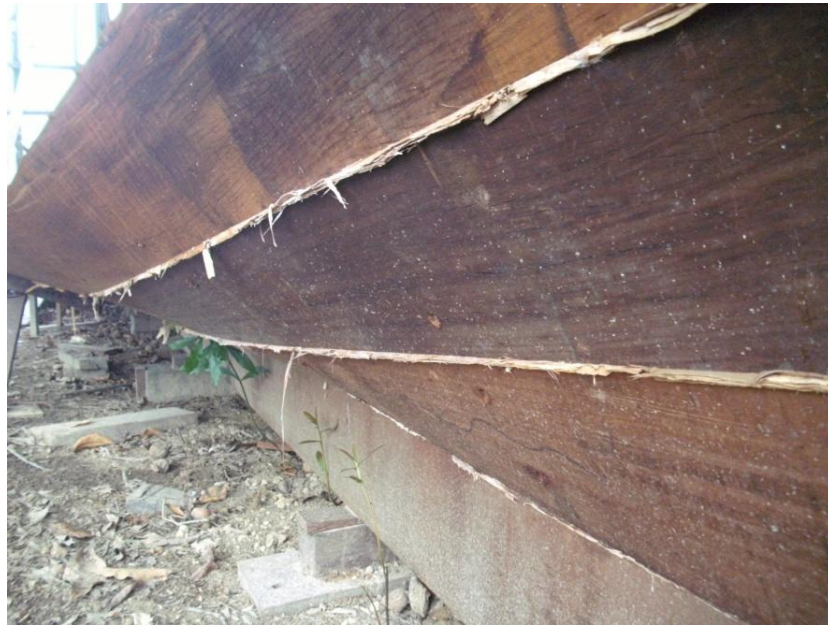
Photo 4.24. Melaleuca bark used to seal planks. Kuala Terengganu.
