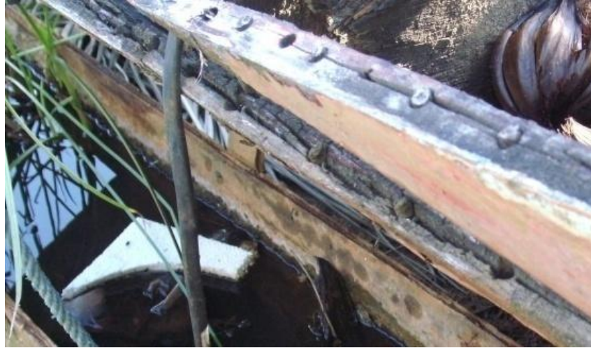
Photo 4.26. Cracked planking through trunnel holes. Kuala Terengganu.
