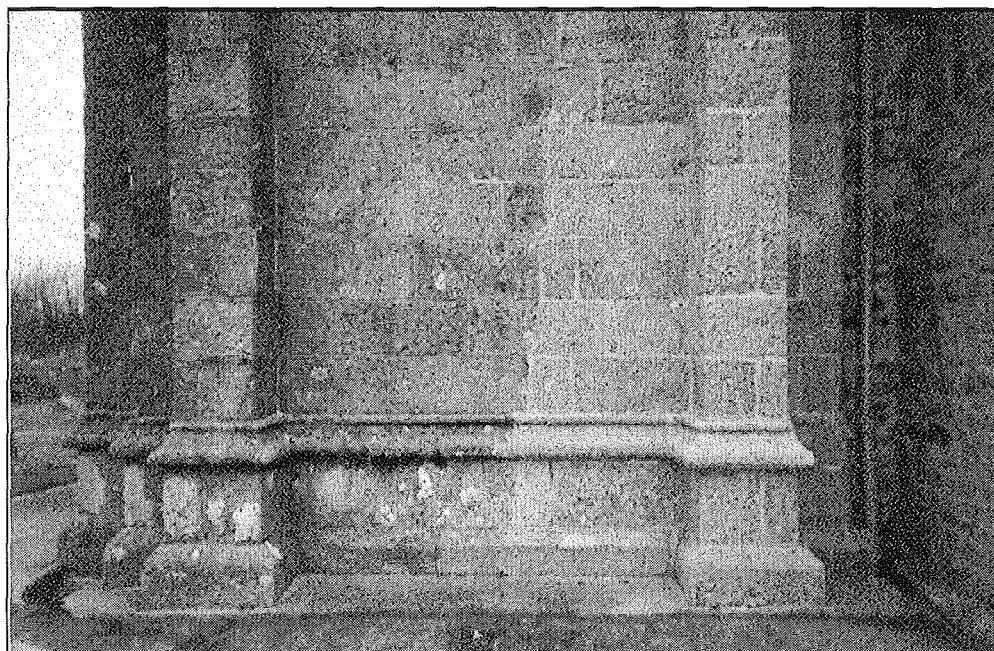
Plate 7.2. Lydford church, south facing wall, showing cleaned area.
