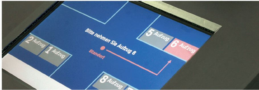
Fig. 4. Destination Selection Control (DSC). The photo (©ThyssenKrupp) shows the indication of the elevator to be taken.
