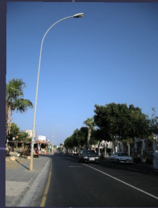
POLE H=5M WITH 70 W H.P. SODIUM
