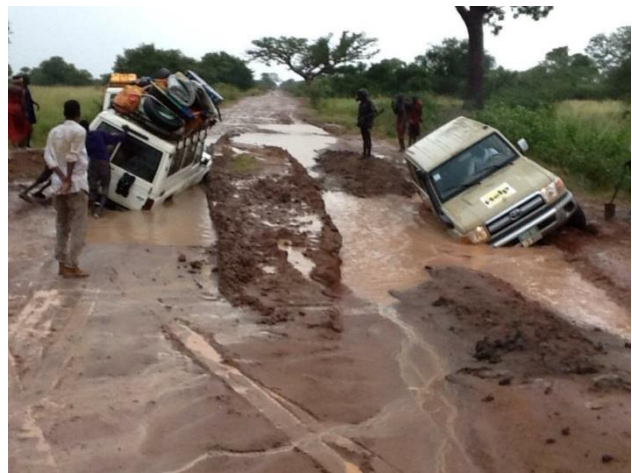
Photo 9 Poor and insecure roads to rural communities showing difficulty of access for social services: Terekeka-Awerial road: Photo by: Gido Lokosang, 16 th Oct 2019.
