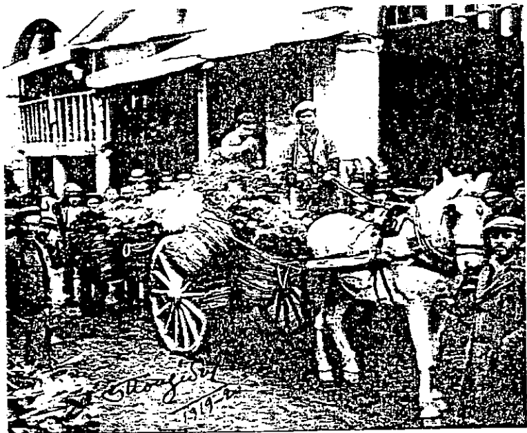
95. The Central market in 1920 (source: ERT, 1992)
