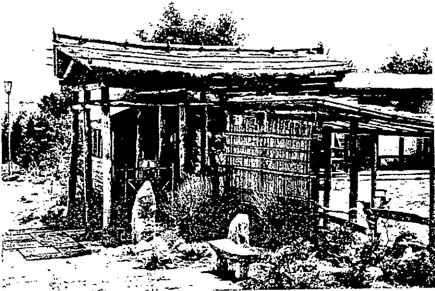
246. Children's playground by D. Pikionis (1965) (source: Pikionis' Works)
