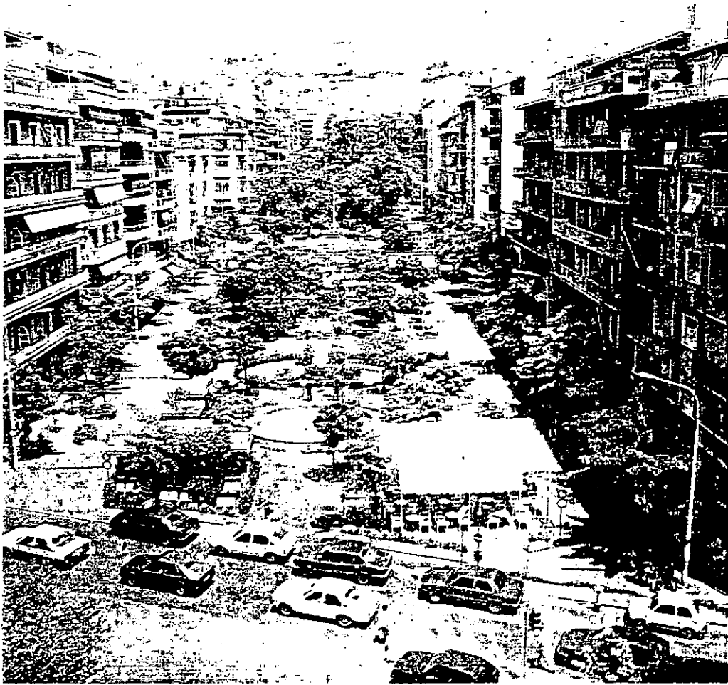
575. Fokionos Negri (1987) (source: Ministry of Environment, Regional Planning and Public Works)
