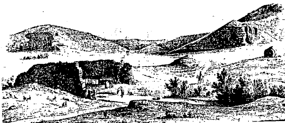
46. The Stadium before its reconstruction, with Ilissos' bridge's ruins (Stademann 1860, source: Biris 1996)
