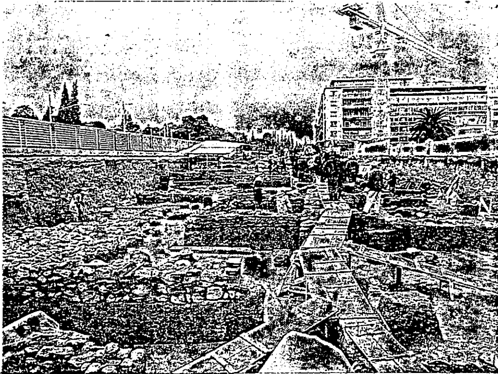
426. Excavations in Syntagma Square for Metro's constructions (1998) (source: author's collection)
