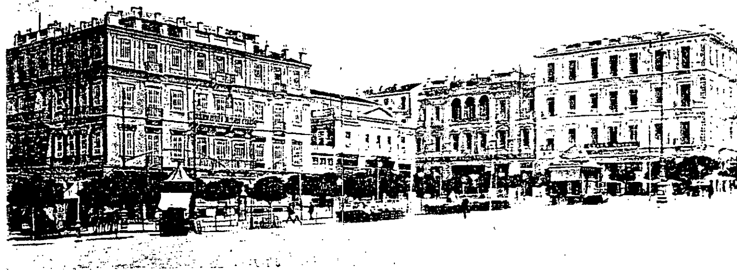
394. Syntagma Square in 1870 with cafés' tables on the lower part (source: Souvenir from Athens)
