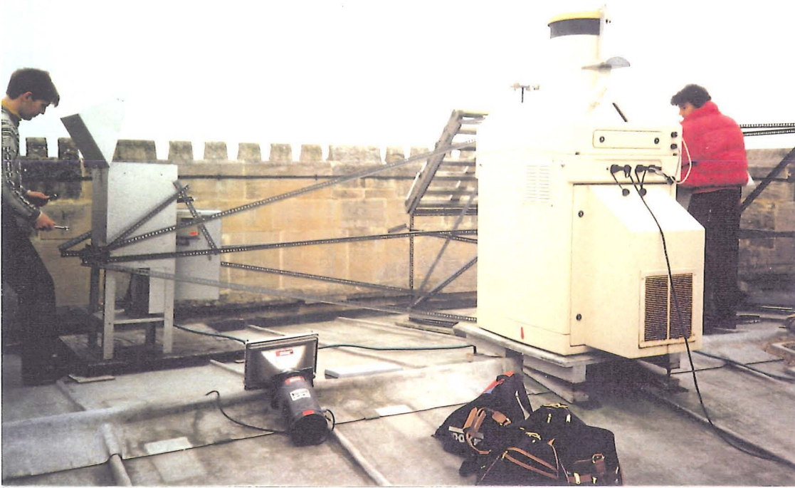
Plate 4.2 (c) Dexion frame restraining the high volume sampler on the north-west tower at Wells Cathedral.
