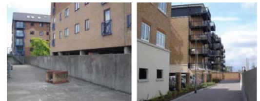
fig03. Flood defences and ground floor parking challenge place-making [8]
