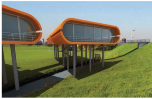
fig06. Paalwoningen 'stilt houses', Haarlemmermeer, Waterstudio (houses in a water-retention area in N.Holland, which have been raised above the floodplain, exploiting a site which would otherwise be uninhabitable).
