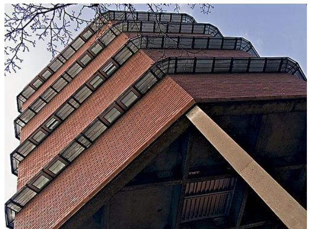
1.4 James Stirling and James Gowan, Leicester University Engineering Building, England (1963)
