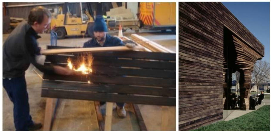
8.4 DSDHA Potters' Fields Park Pavillion, London (2008) Charring and finished surface
