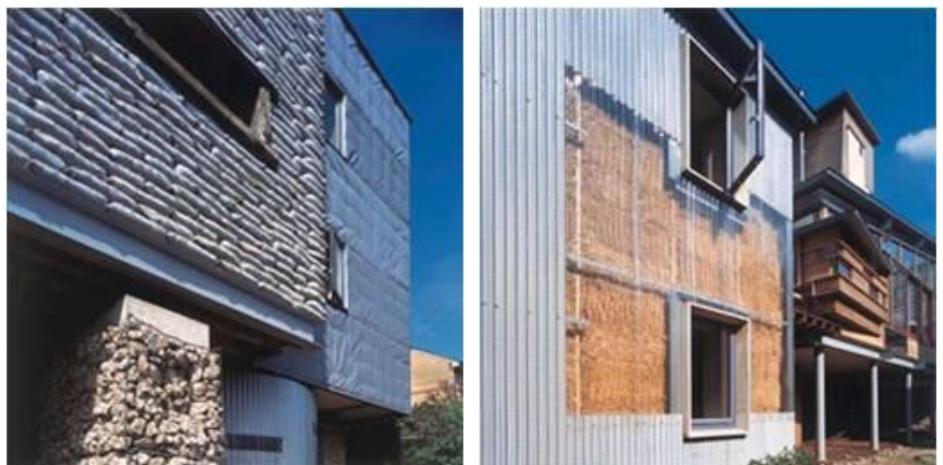
8.6 Sarah Wigglesworth Architects, Stock Orchard Street house, London (2004) uses of materials
