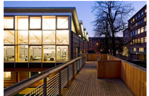
3.2 Mole Architects, Stressed Skin Roof at School of Architecture, Cambridge (2006)
