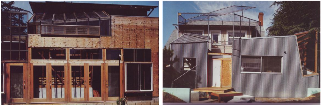
8.11 Frank Gehry, Gehry House, Santa Monica, California (1978)
