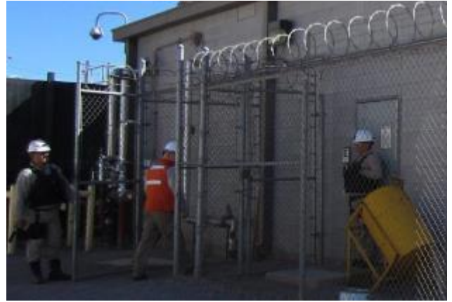
Figure 17: Refinery access control
