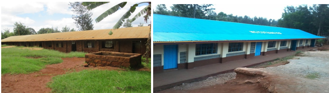
Photo 26: Baraka classrooms, May 2016 Photo 27: Refurbished Baraka classrooms, April 2017
