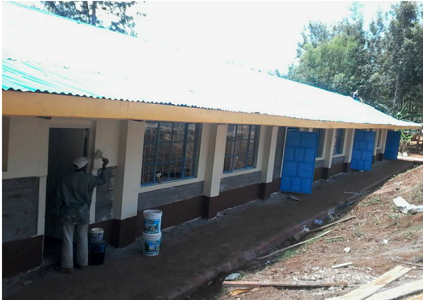
Photo 22: Baraka classroom refurbishment in April 2017
