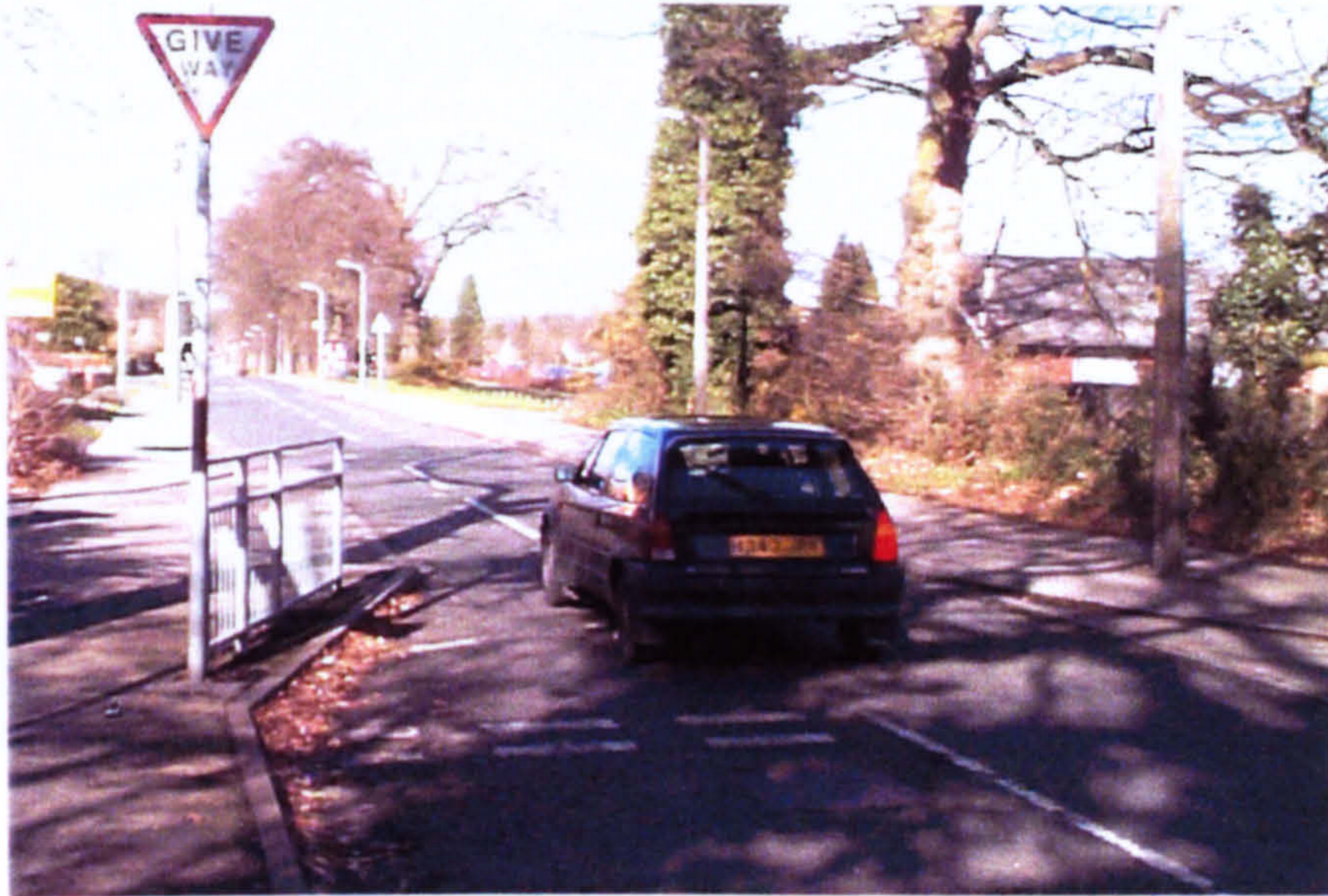
Plate 5.7 Build-out: Owlsmoor Road, Sandhurst.
