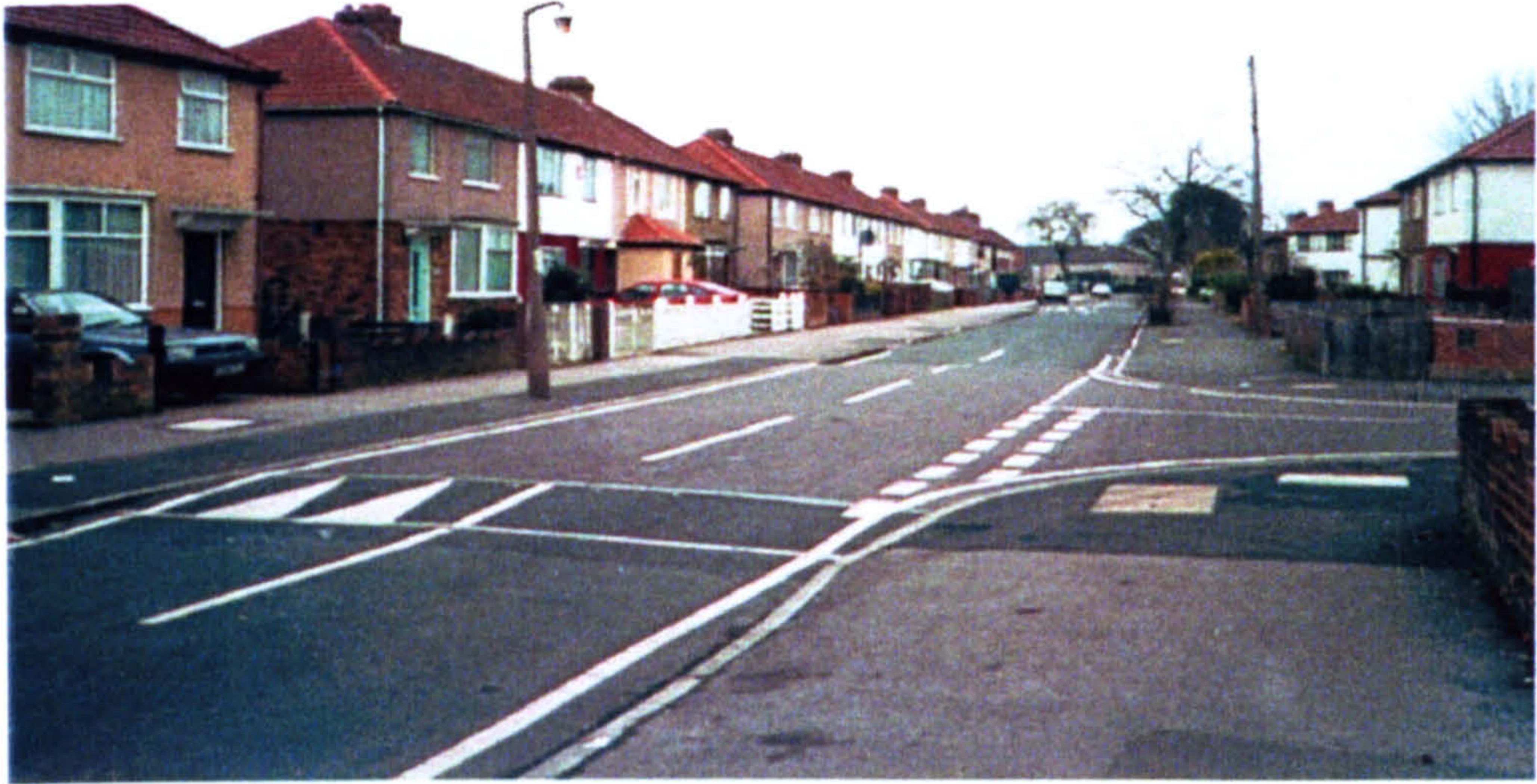
Plate 5.5 Raised junction: Carlton Road, Slough.
