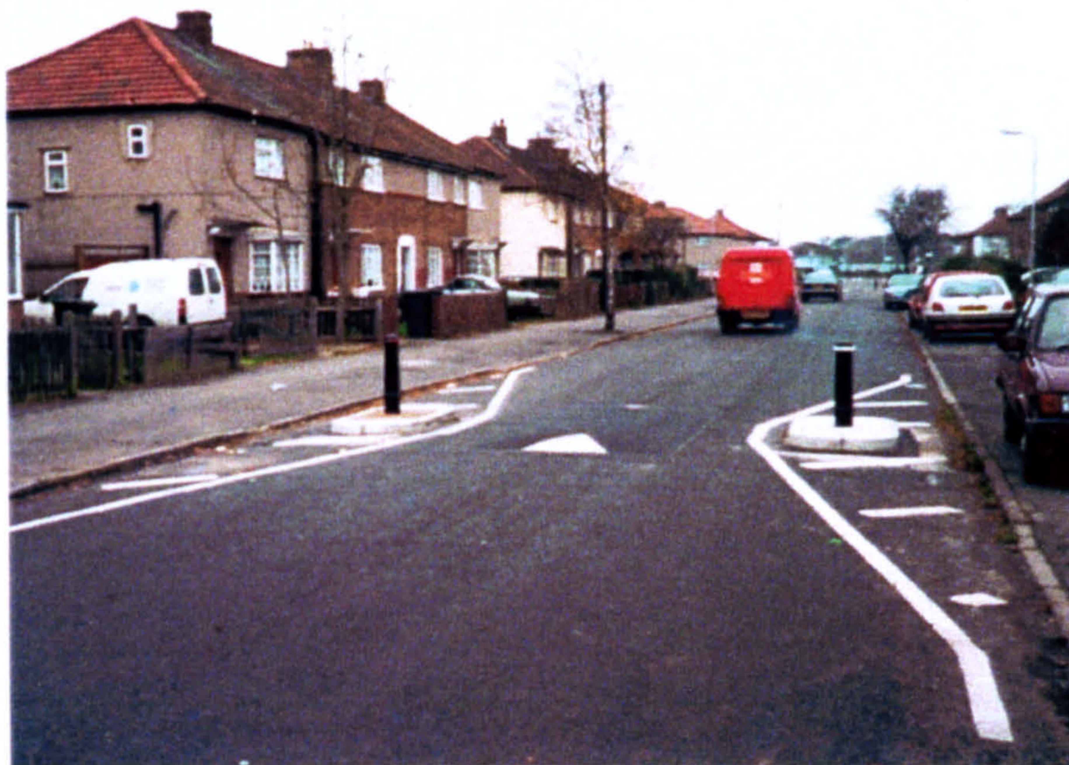
Plate 5.4 Combined pinch point and speed cushion: Broadmark Road, Slough.
