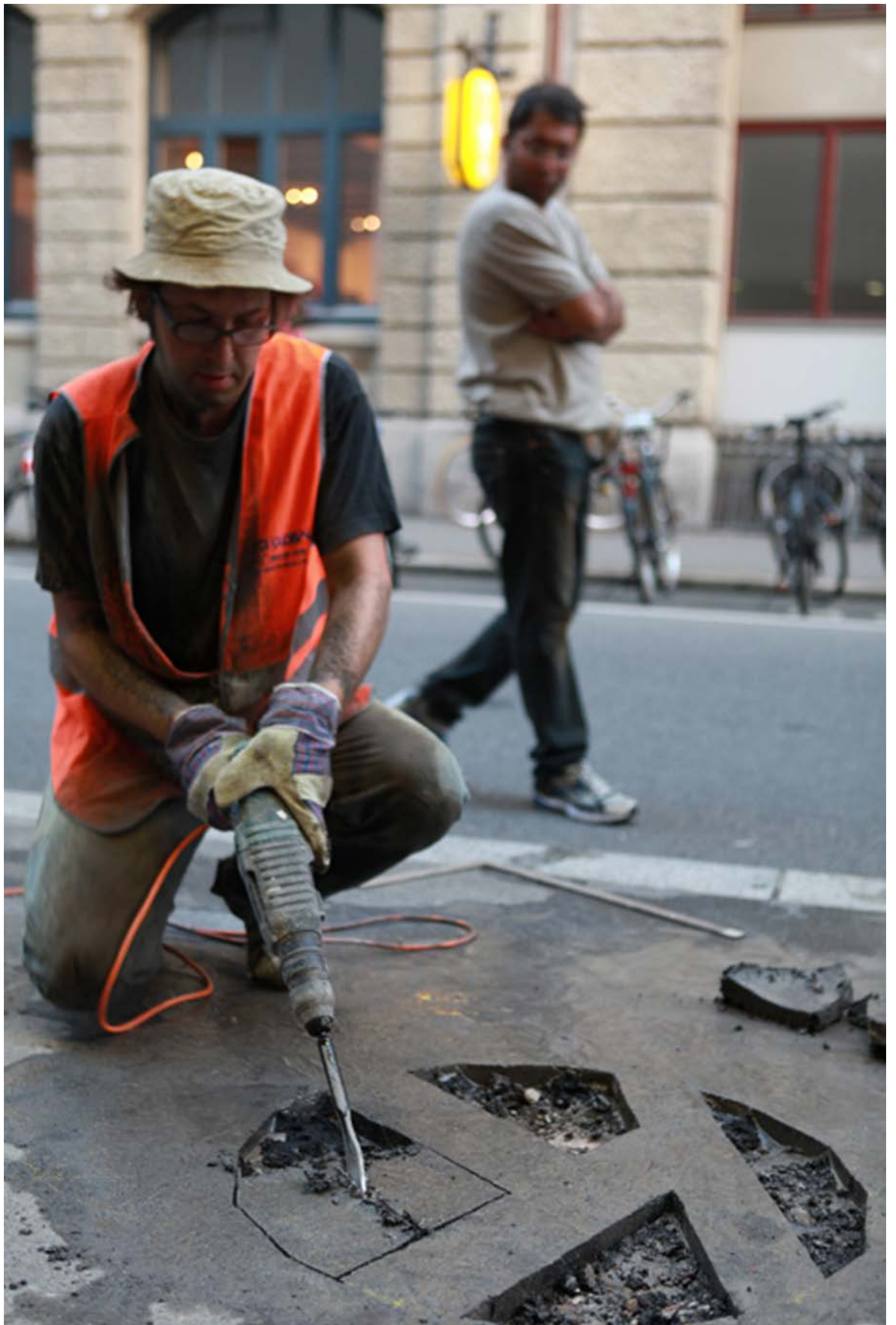
Figure 9 Hardliz, R., Exit Strategy (Bourbaki) , drilling the logo of Kunsthalle Luzern into the sidewalk refilling it with asphalt, Luzern, 2011, photo: Beate Engel, 2011
