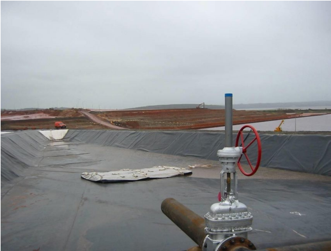
Figure 49 Inlet filling valve to one Demonstration cell 2007
