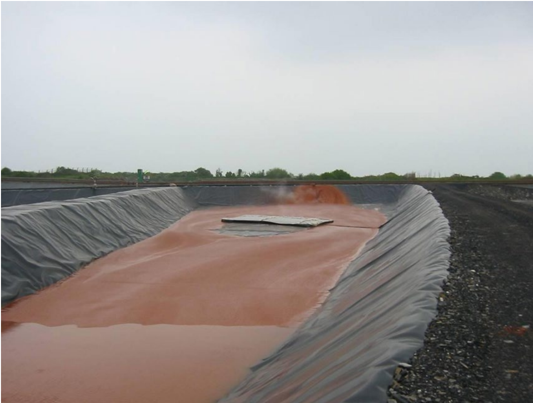
Figure 51 Bauxite Residue deposited after first fill 2007
