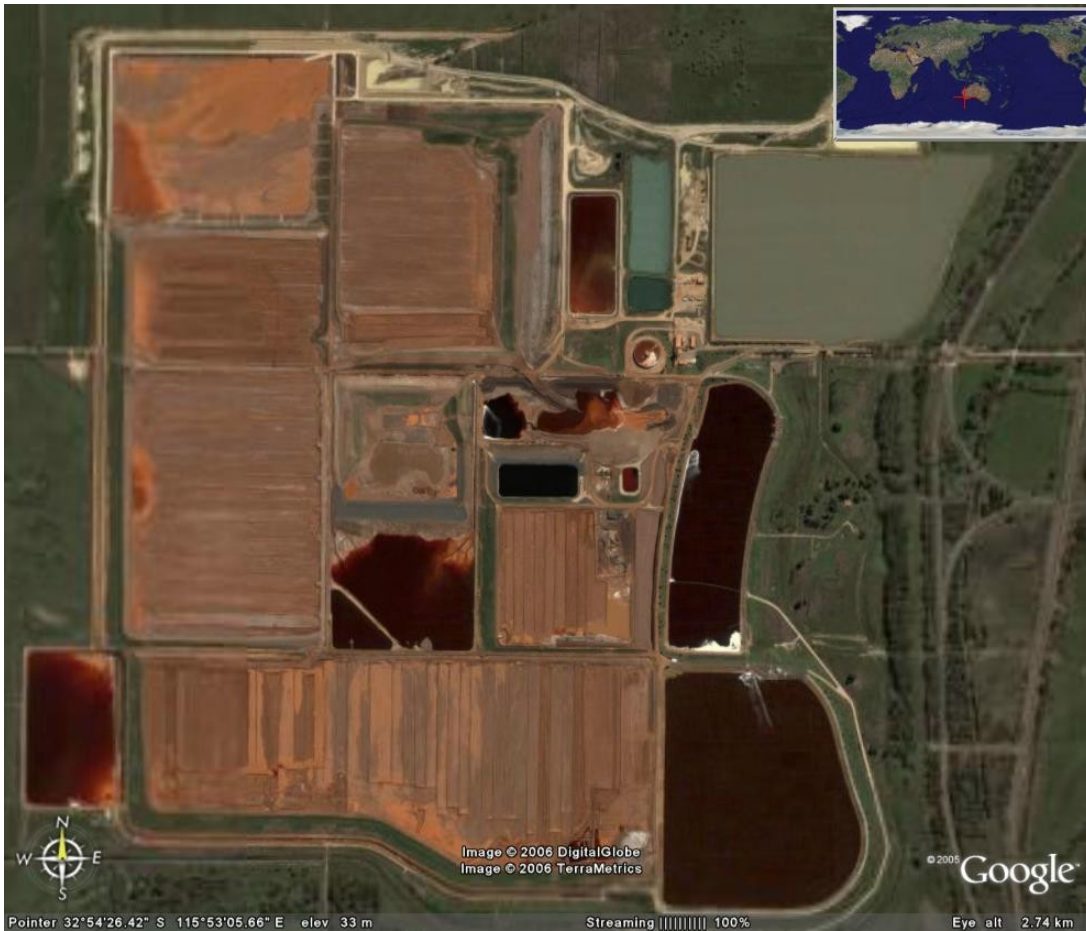
Figure 8 Wagerup Residue Disposal Facility (Google, 2007)
