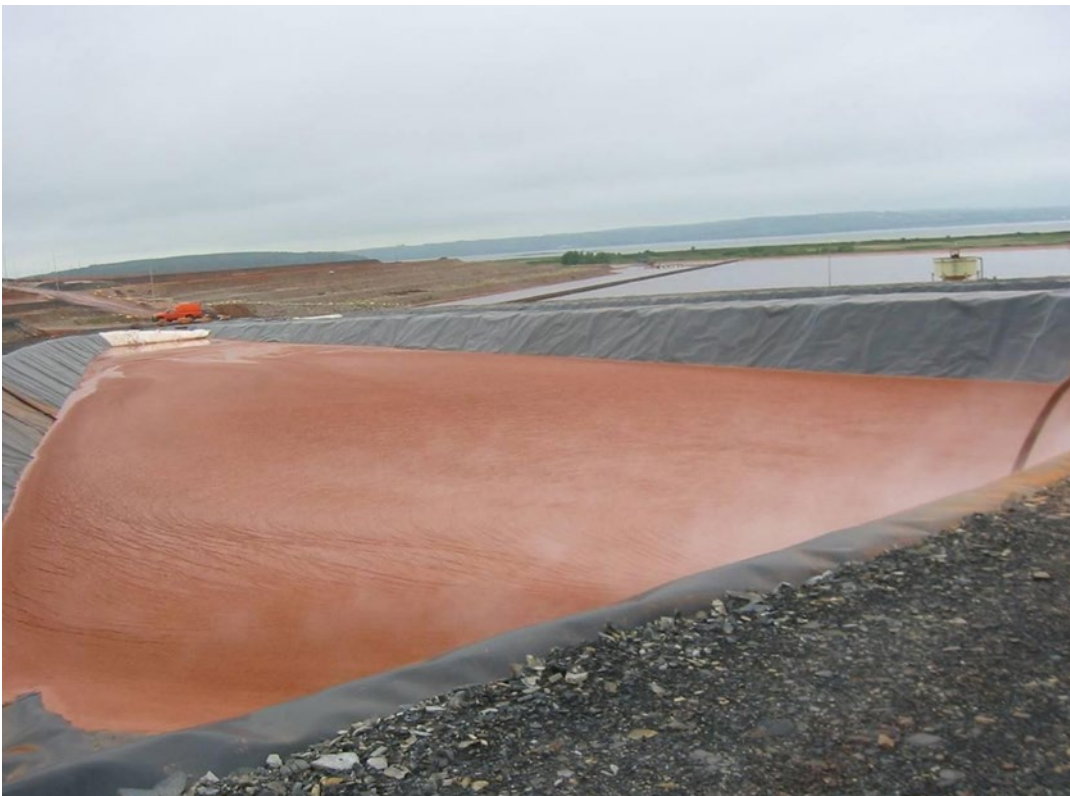
Figure 52 Second fill into Demonstration cell 2007
