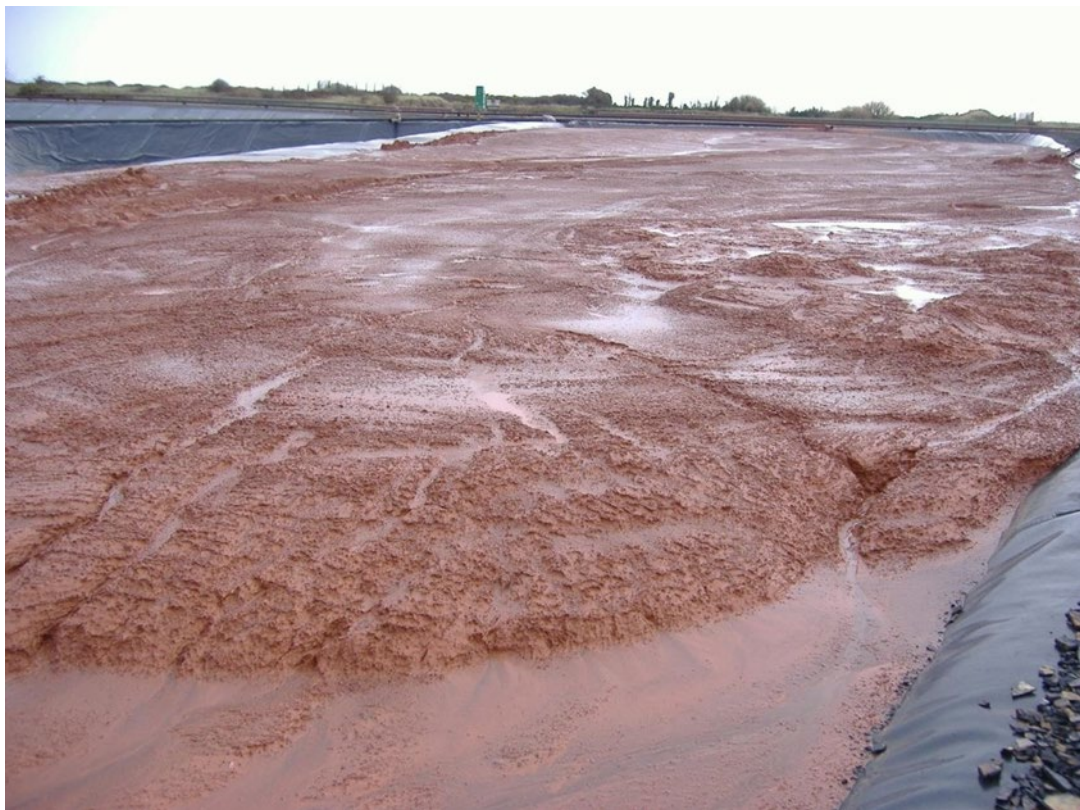
Figure 54 Demonstration Cell filled with red mud 2007
