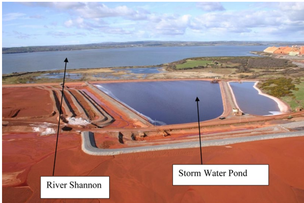
Figure 4 Embankments on east side of the B.R.D.A. and Storm Water Pond. 2006
