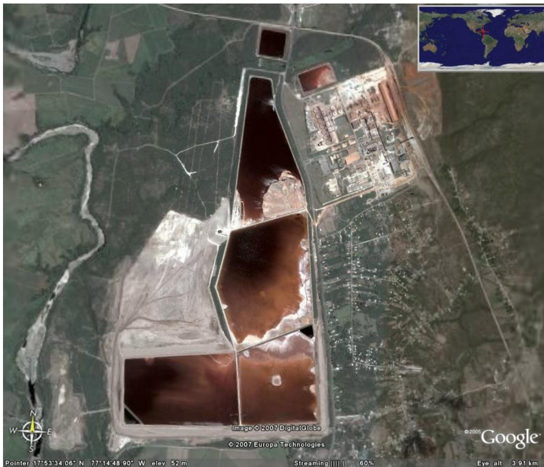
Figure 13 Overview of Jamalco Residue Disposal Facilities (Google, 2007).
