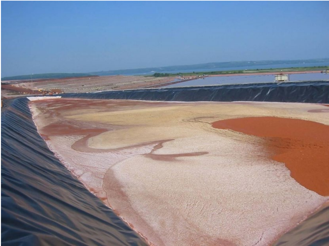
Figure 53 Level in cell after 3rd fill (white colour is evidence of soda) 2007
