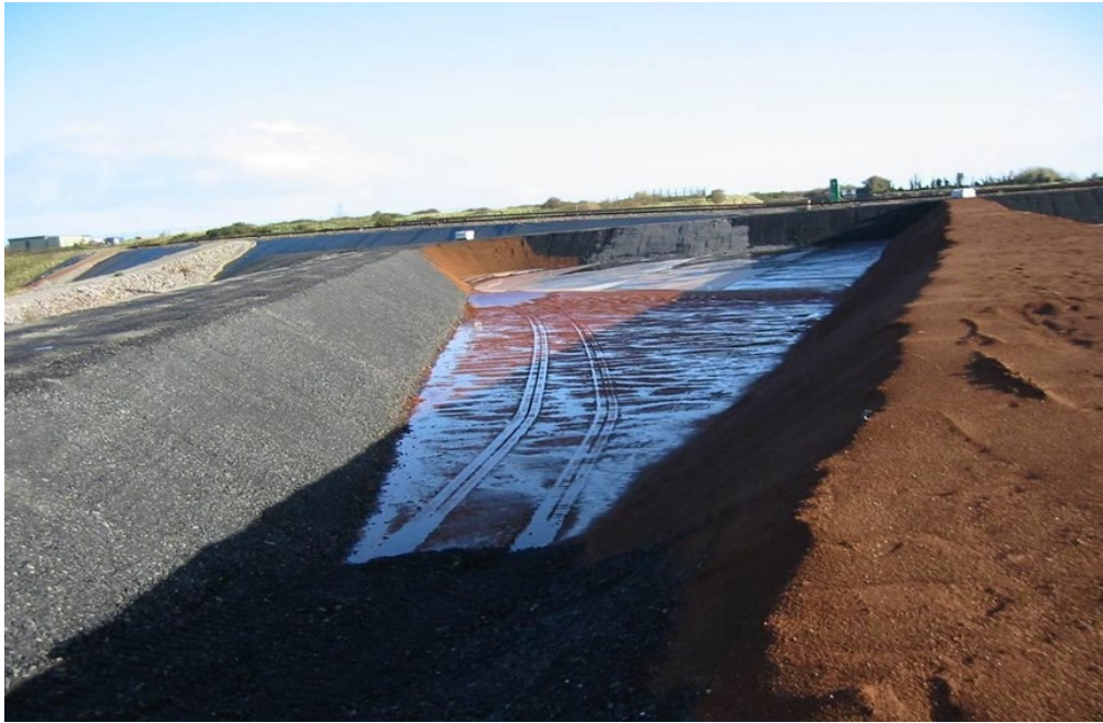
Figure 47 One Cell before liner was installed, sand and rock only 2006
