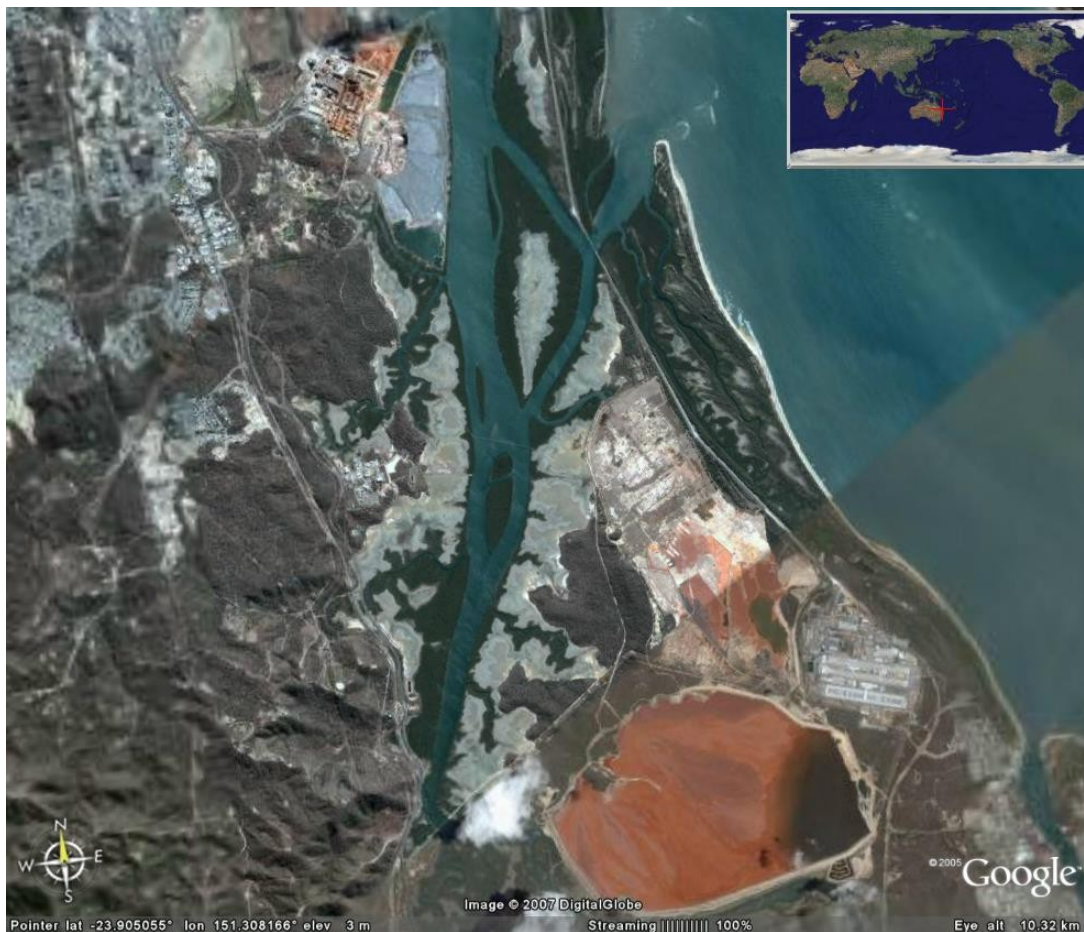
Figure 3 General arrangement of QAL facilities at Gladstone, Queensland (Google, 2007).
